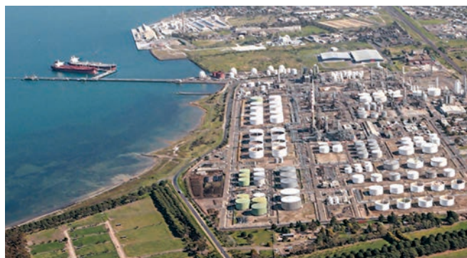
FIG. 1. The Geelong refinery in Australia.
