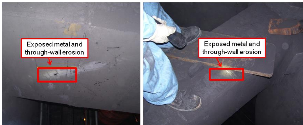
Figure 4. Erosion and wall holing: short side of crossover (left), top side of crossover (right)
