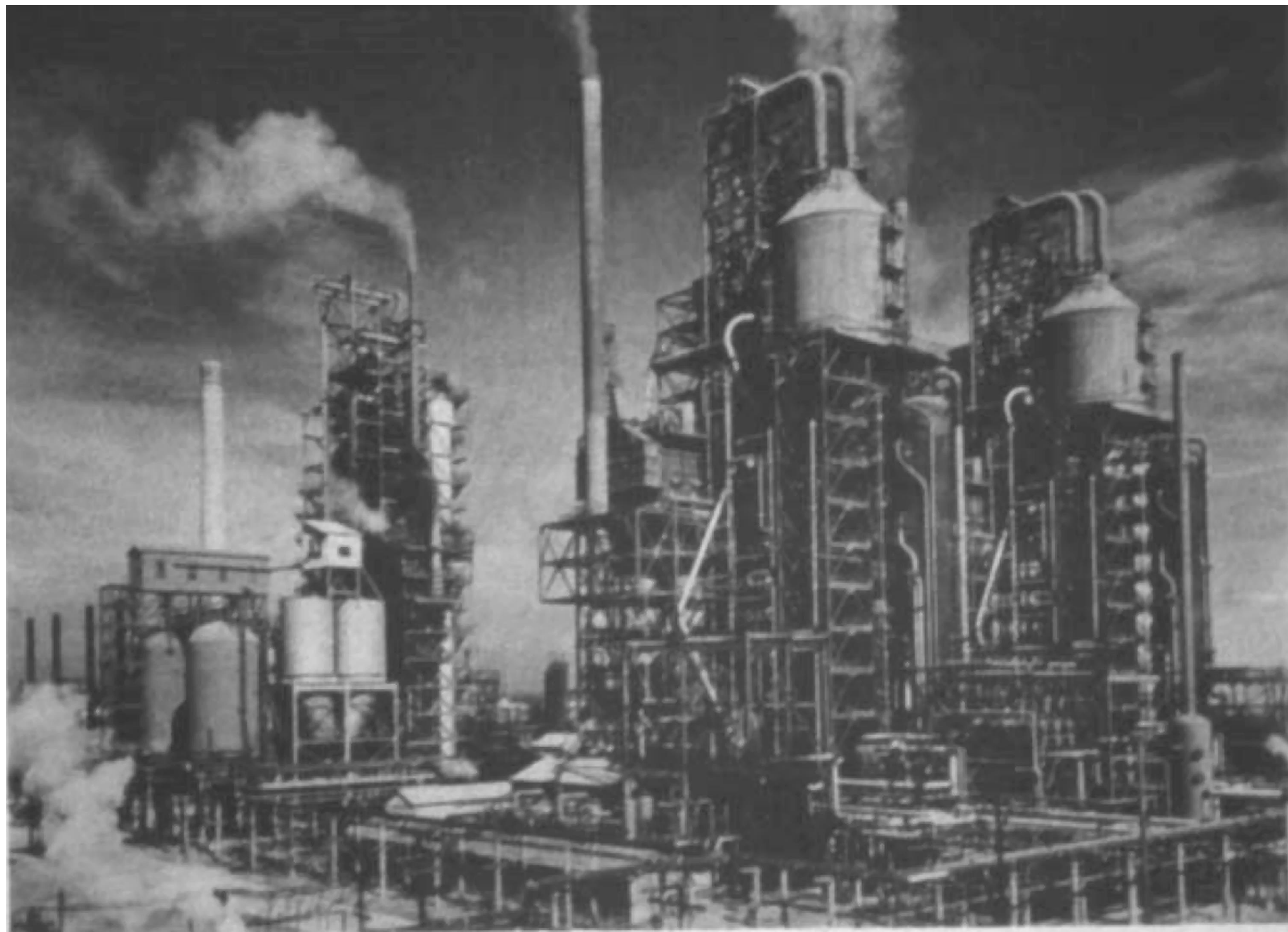
EXXON BATON ROUGE MODEL I AND II FCC'S MODEL I IS ON THE LEFT MODEL II UNITS ARE ON THE RIGHT
